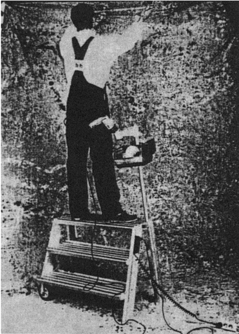
Figure 6. The new working-trestle
