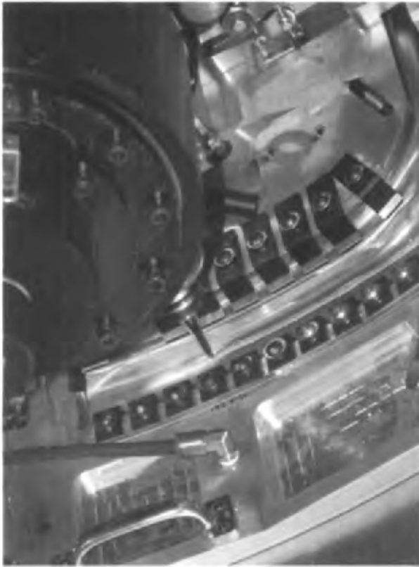
Fig. 7C13i-1 Friction stir welding of aluminum aircraft skin to frame members. Note the clamping devices used to withstand the separation force of the probe of the welding tool. (Photo courtesy Eclipse Aviation.)
