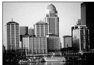
Fig. 2.41. World's Largest Heat Pump System in Louisville, KY.
